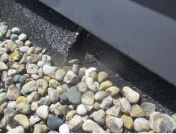
Photo #19 Typical view of open flashing membrane
