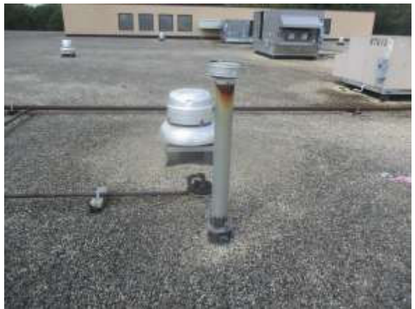
Photo #4 Typical view of roof vents and pipe penetrations
