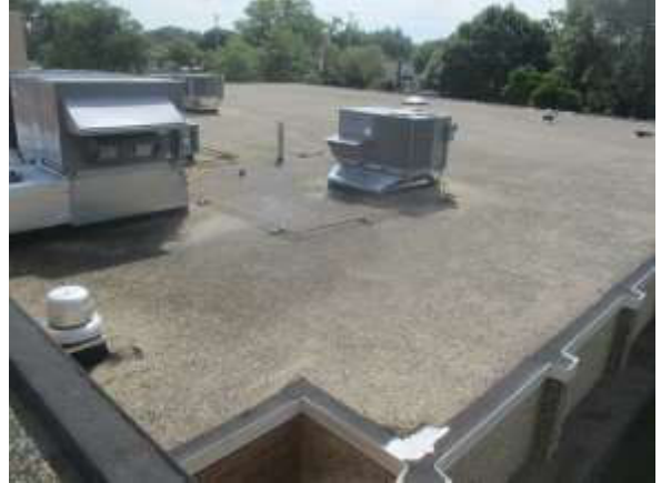
Photo #14 Overall view of the office roof
