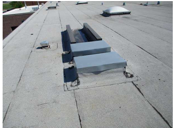
Photo #2 View of existing curb from previously removed mounted equipment
