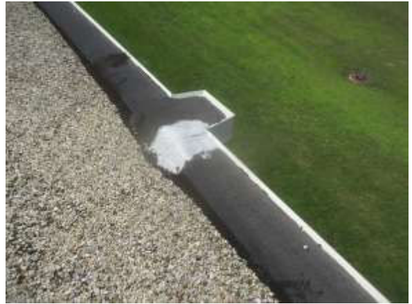
Photo #16 Typical view of perimeter edge repairs
