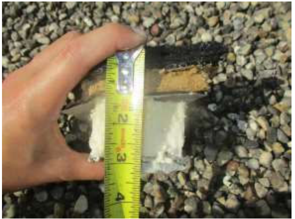
Photo #22 Typical view of roof system
