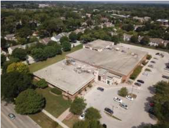
Photo #1 Overall view of building
