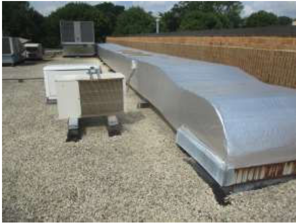
Photo #15 Typical view of ductwork.
