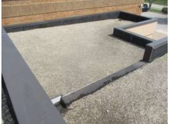
Photo #18 View of lower roof near entrance.
