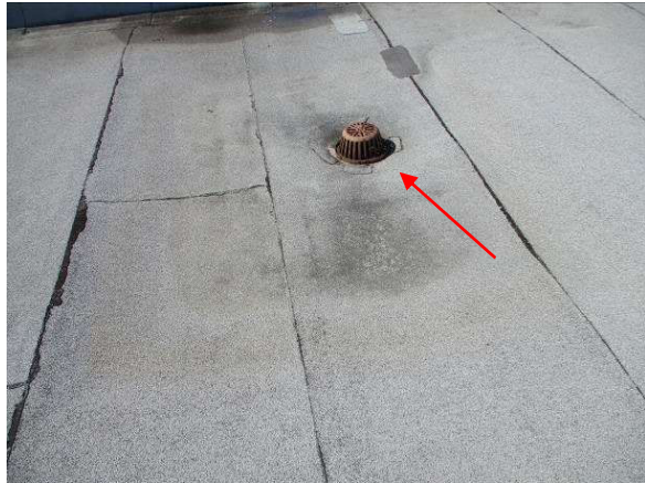
Photo #1 Overall view of sump and roof drain
