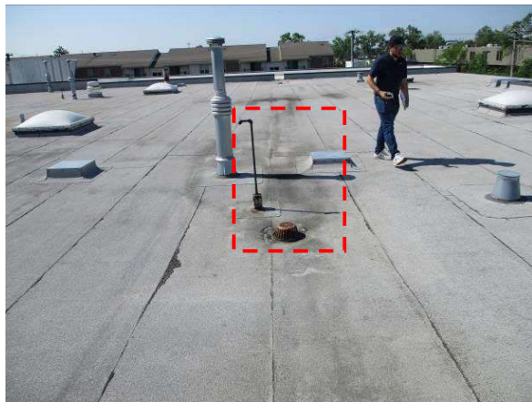
Photo #3 View of previous membrane seam repair
