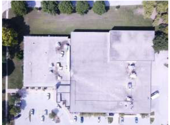
Photo #2 Overall view of roof areas from above
