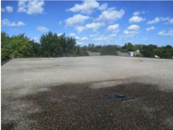
Photo #13 Overall view of gymnasium roof
