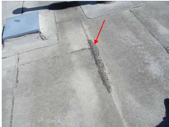
Photo #3 View of previous membrane seam repair
