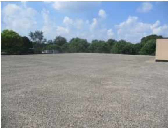
Photo #3 Overall view of the Main Roof gravel surface membrane.
